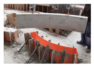
For a building renovation, NOWLAB helped construction company Geiger to reduce costs and time in creating large concrete casting molds.
